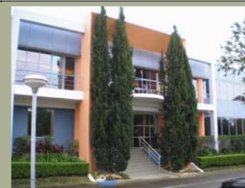
219 North Rocks Road, North Rocks NSW
