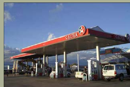
Caltex Service Centre Portfolio, Goondiwindi/Emerald/Stanthorpe QLD
