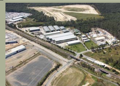
63 Burnside Rd, Stapylton QLD
